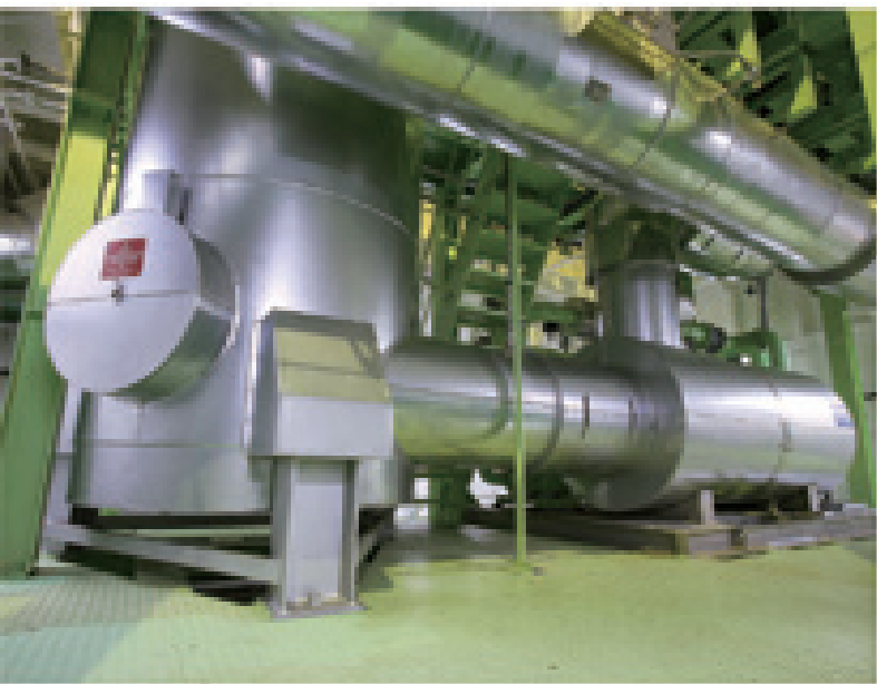
▲ Selective Catalytic Reduction Reactor (SCR)
